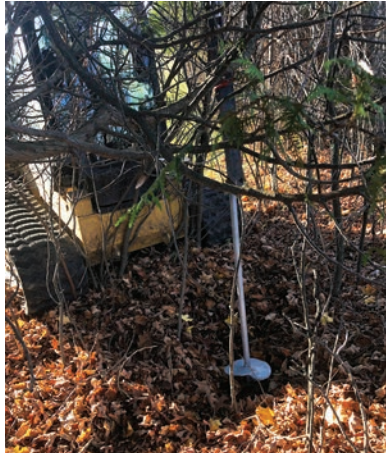
Mike Jorgenson uses our grant funded skid steer to auger in a down-guy anchor.
