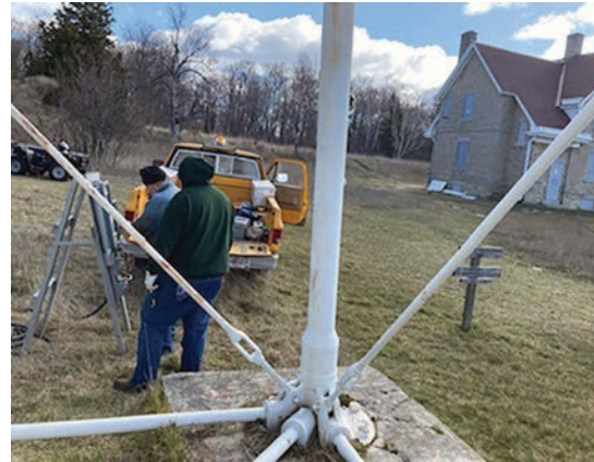
Installing temporary service at the 1896 rear range light.
