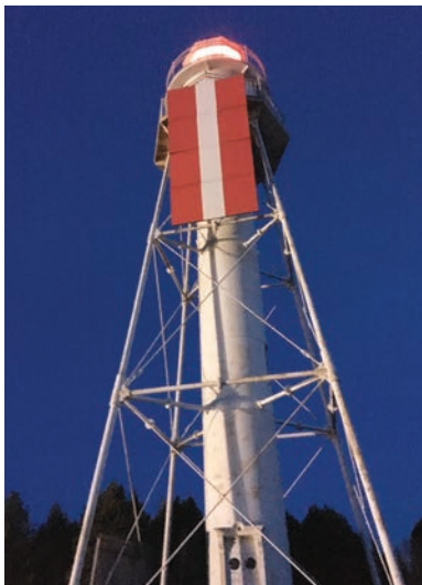
The 1896 rear range light on Plum Island prior to restoration.
