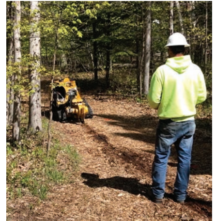
Karcz’s cable-sneaking machine installing 1-inch conduit for fiber.
