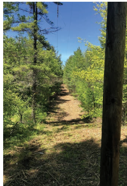
Right-of-way cleared using the skid loader purchased with fiber grant.
