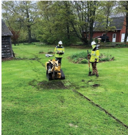
Karcz’s cable-sneaking machine installing 1-inch conduit for fiber.
