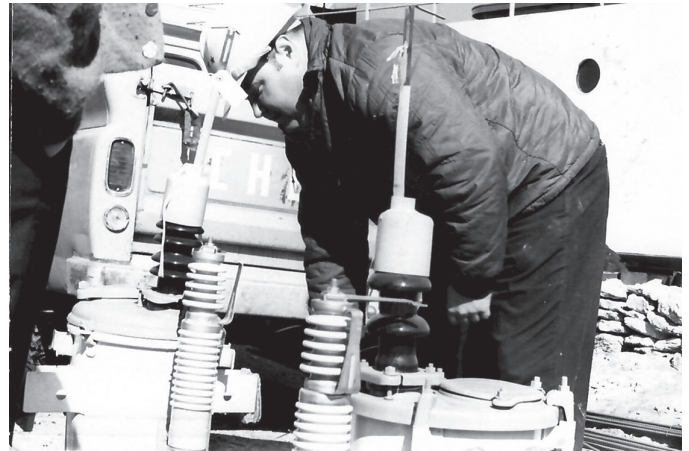
Irwing "Henry" Nelson inspecting rebuilt transformers delivered from WECA/RESCO in 1969
