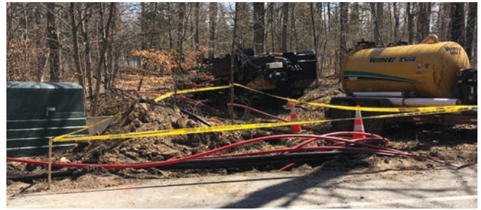
The boring machine got quite a workout in the rocky ground.
