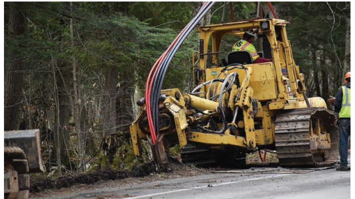
KS vibratory cable plow arriving on the Madonna (truck driver and operator's first time on a ferry), and at work below.
