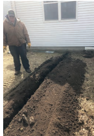
Your crew and Quantum working together to install conduit for a fiber link between the Bethel Church and parsonage.
