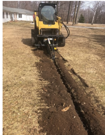
Your crew and Quantum working together to install conduit for a fiber link between the Bethel Church and parsonage.
