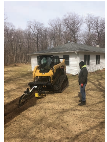
Your crew and Quantum working together to install conduit for a fiber link between the Bethel Church and parsonage.
