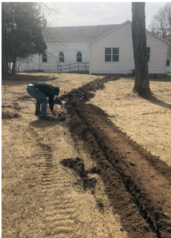
Your crew and Quantum working together to install conduit for a fiber link between the Bethel Church and parsonage.
