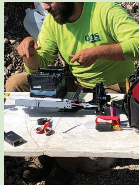
Nsight contractor QOS splices cable on the south side of Plum Island.
