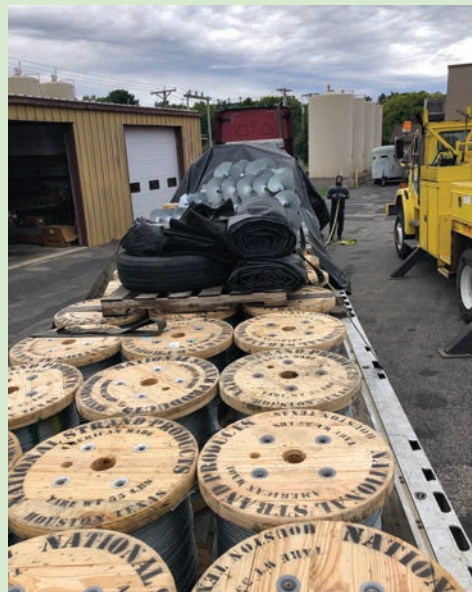
Using the digger derrick to unload reels of cable.
