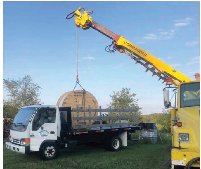
The first 20,000-foot reel of 96 strand fiber are unloaded at the cooperative.
