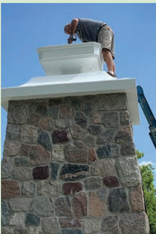
Left to right: Dave Llewellyn drills the once planter, now eagle base for a pin while Tom Bloch (in photo, second from left) steadies the ladder; the eagle is tipped down for a stabilizing pin; the eagle's base is drilled for the stabilizing pin.
