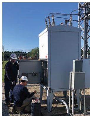
Top photo: Eaton personnel on site for substation breaker maintenance. Left: Mike Jorgenson isolates the breaker from the system. Right: Eaton personnel prepare for testing and preventive maintenance.
