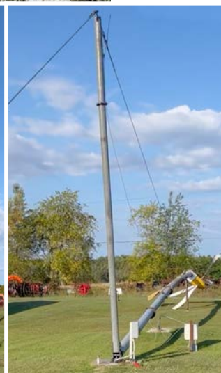
Inset above: Wind generator (seagull killer) goes down—quickly—after snapping the anchor from the concrete.
