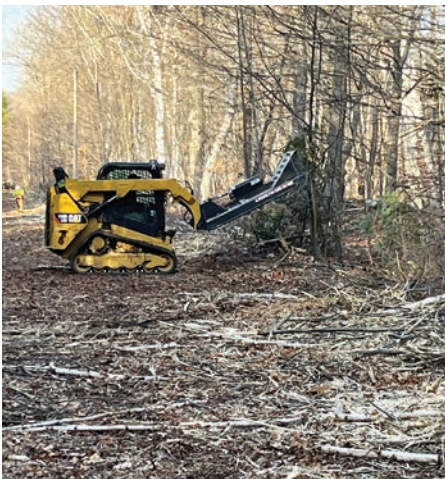
Mike brushing the right-of-way.
