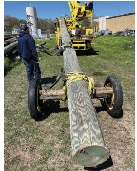
An 80-foot pole is delivered to the Ferry Dock area for a third small cell.
